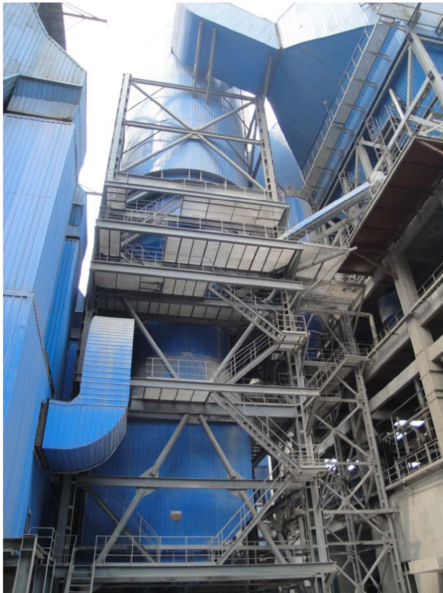
Figure 17 - Matou Power Plant CFB System
