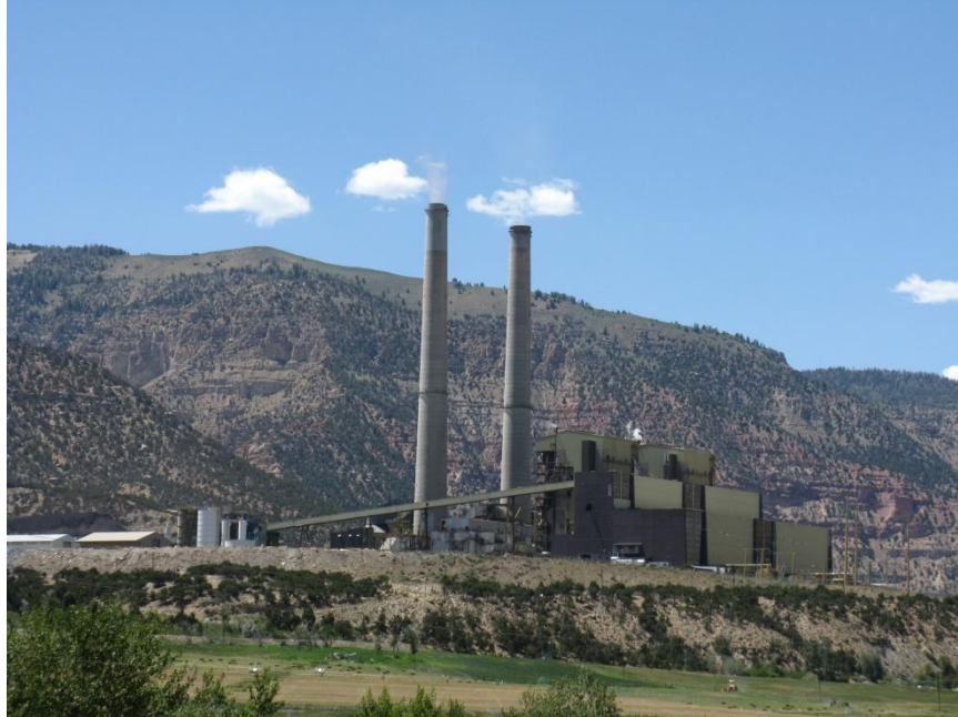
Picture 2: Huntington Power Station
