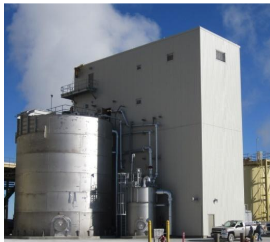
Picture 4: New Hunter Dewatering Building
