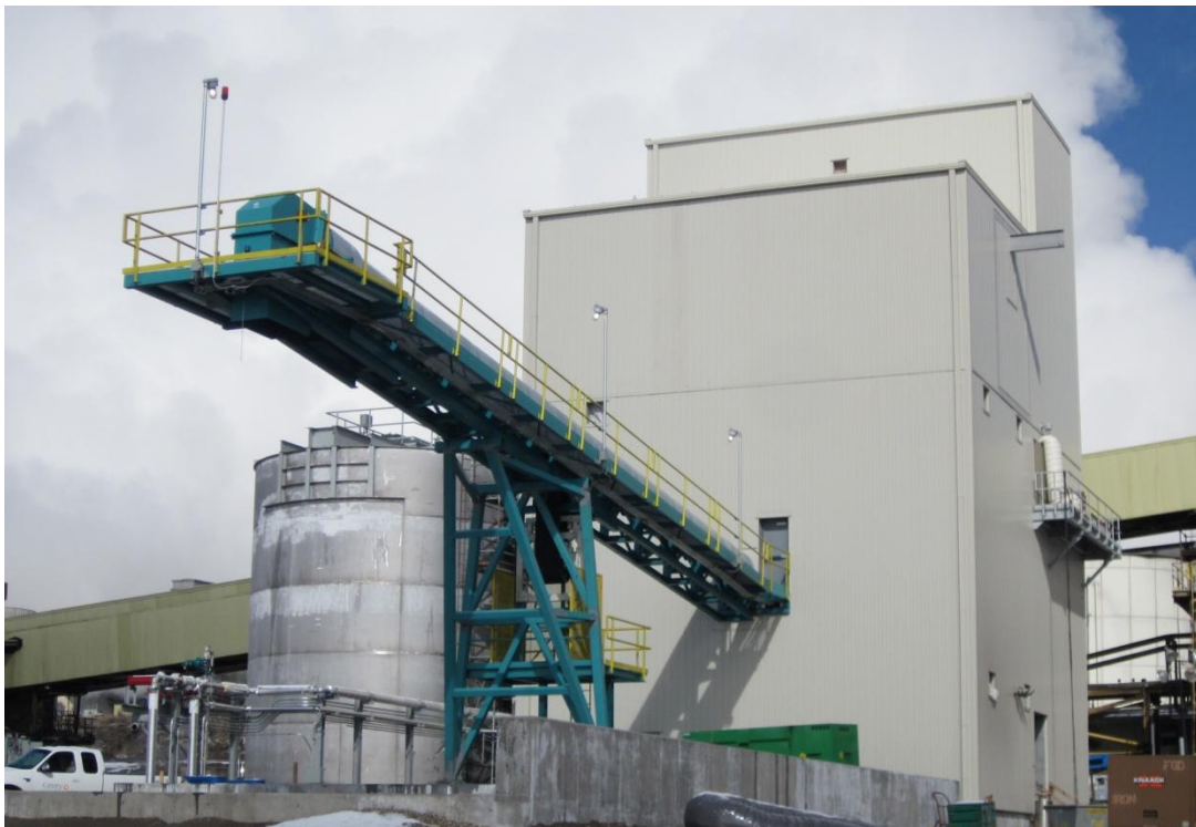
Picture 3: New Huntington Dewatering Building
