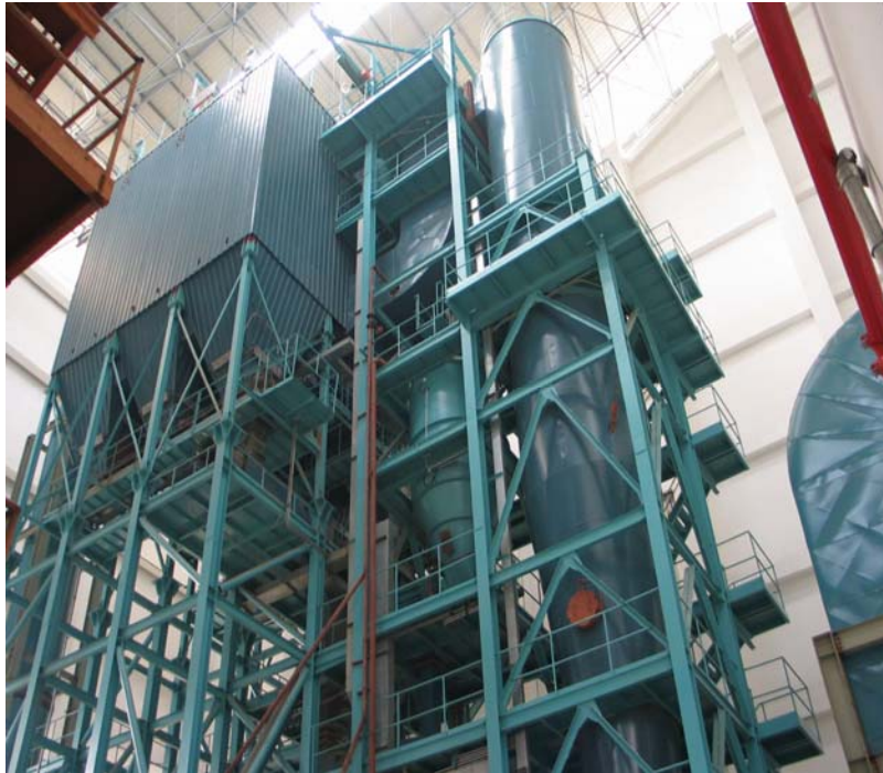
Figure 14 - Wangneng Waste to Energy Power Plant
